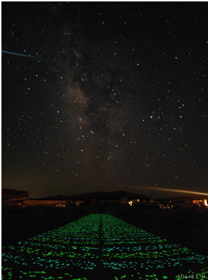
Footpath in the B'eerot campground, with embedded solar-charged resin-based glow stones lights up the way between the tent area and public toilets/shower area. No additional lights are required. Photo: Juliet H., INPA.
